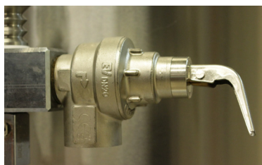
Fig. 0-42 Safety valve open
